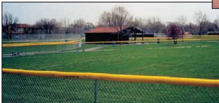
Safety takes effort: (above) Adding protective tubing to fence tops reduces risk of players being injured reaching for home-run balls; (top right) bleachers are more safe with handrails and back guards; (below) ball returns help get balls into play safely; (bottom) and safety bases reduce sliding injuries.
